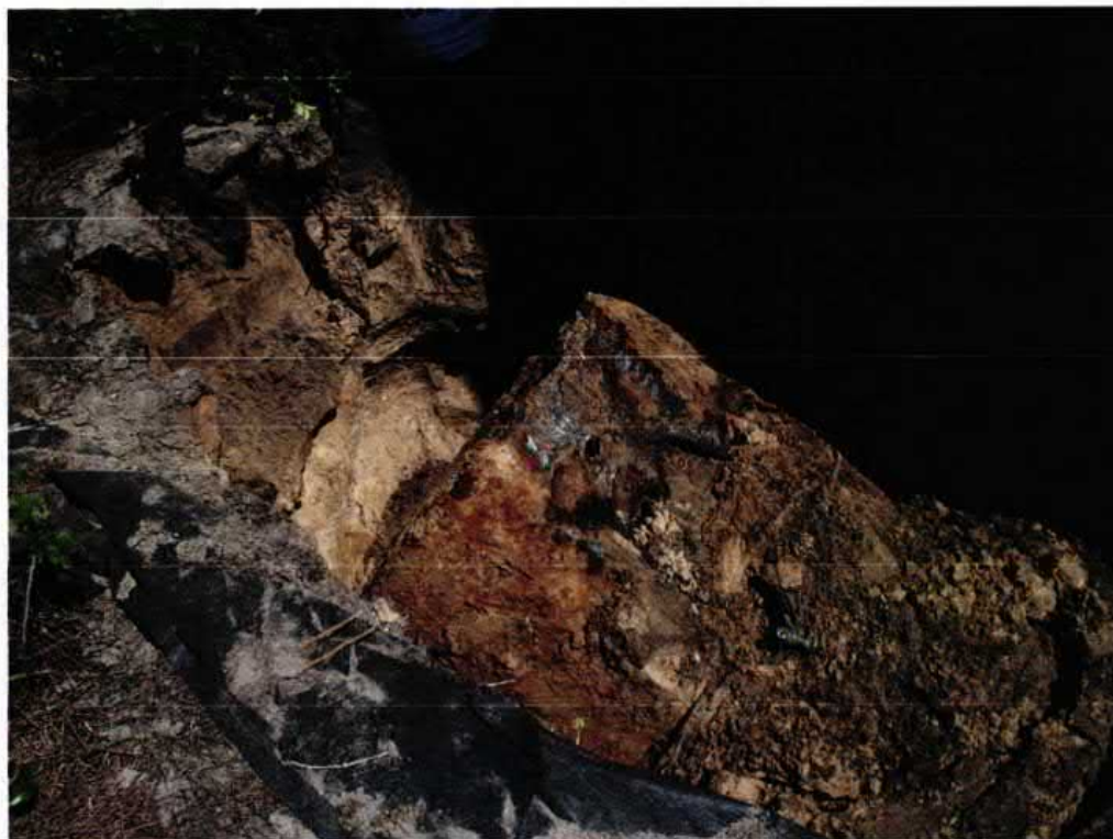
Picture 2: UST 733Bluebell prior to removal from excavation.
